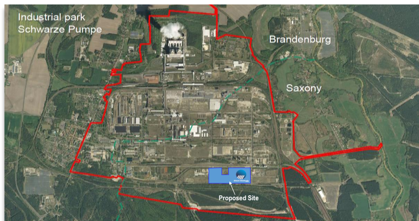
Figure 2.6 Silumina Anodes™ site in Schmarze Pumpe industrial site
