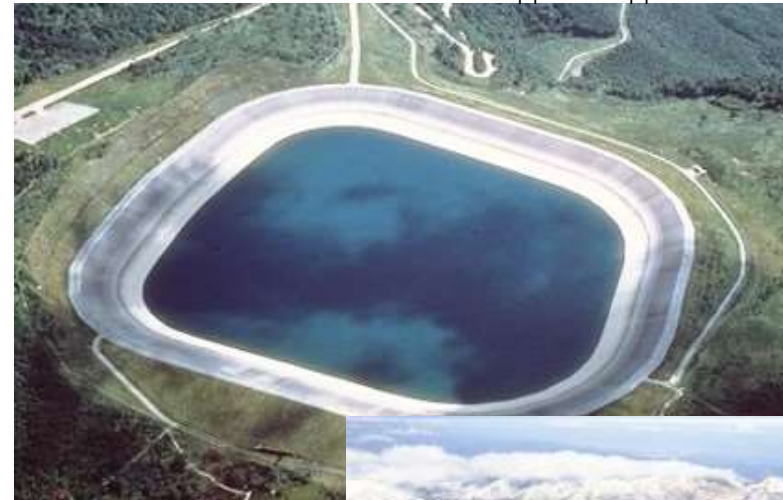
Numappara – upper reservoir
