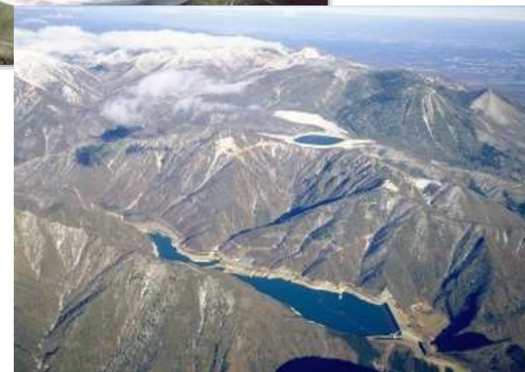
J-POWER'S 675MW Numappara Pumped Storage Hydro Project (1973)
