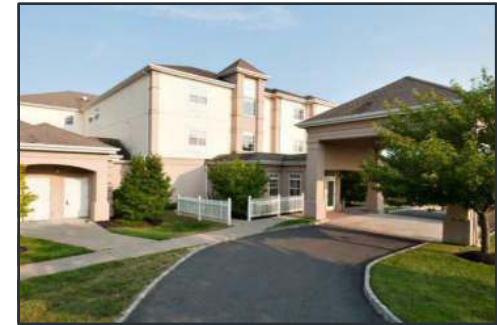
Bear Creek Assisted Living, West Windsor, NJ
