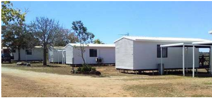
Figure 17(b): Refurbished accommodation cabins at Top Camp
