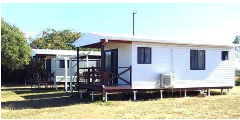
Figure 17(a): Refurbished accommodation cabins at Top Camp
