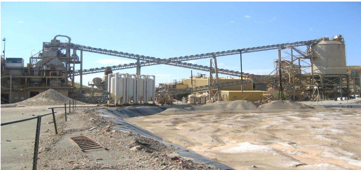
Figure 4: Bamboo Creek Processing Plant
