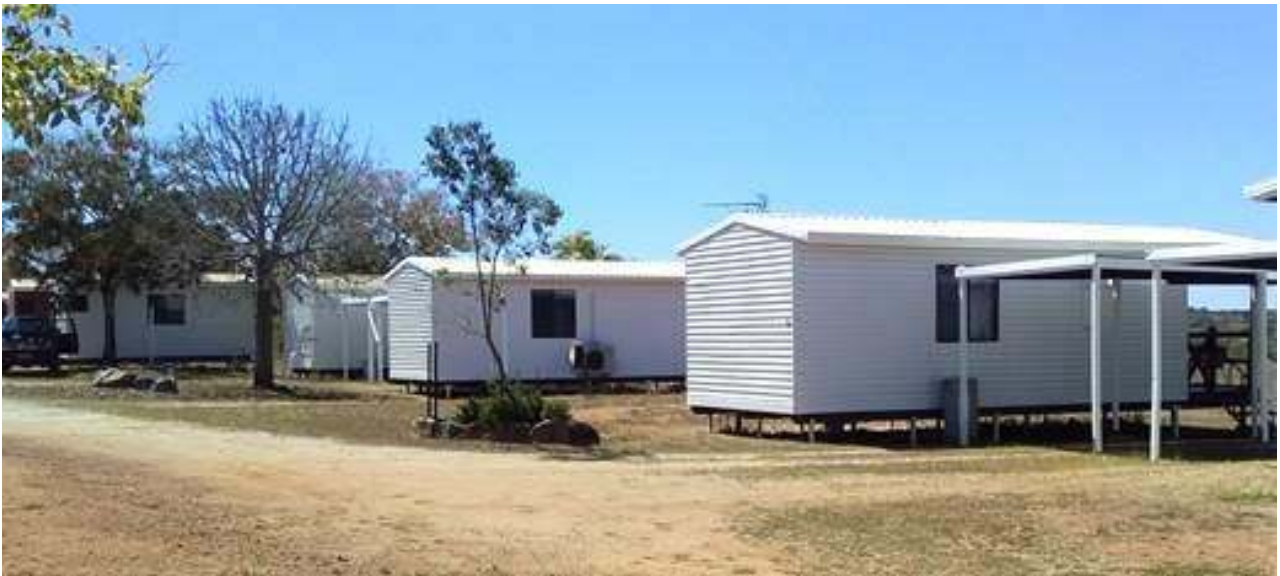
Figure 18b: Refurbished accommodation cabins at Top Camp
