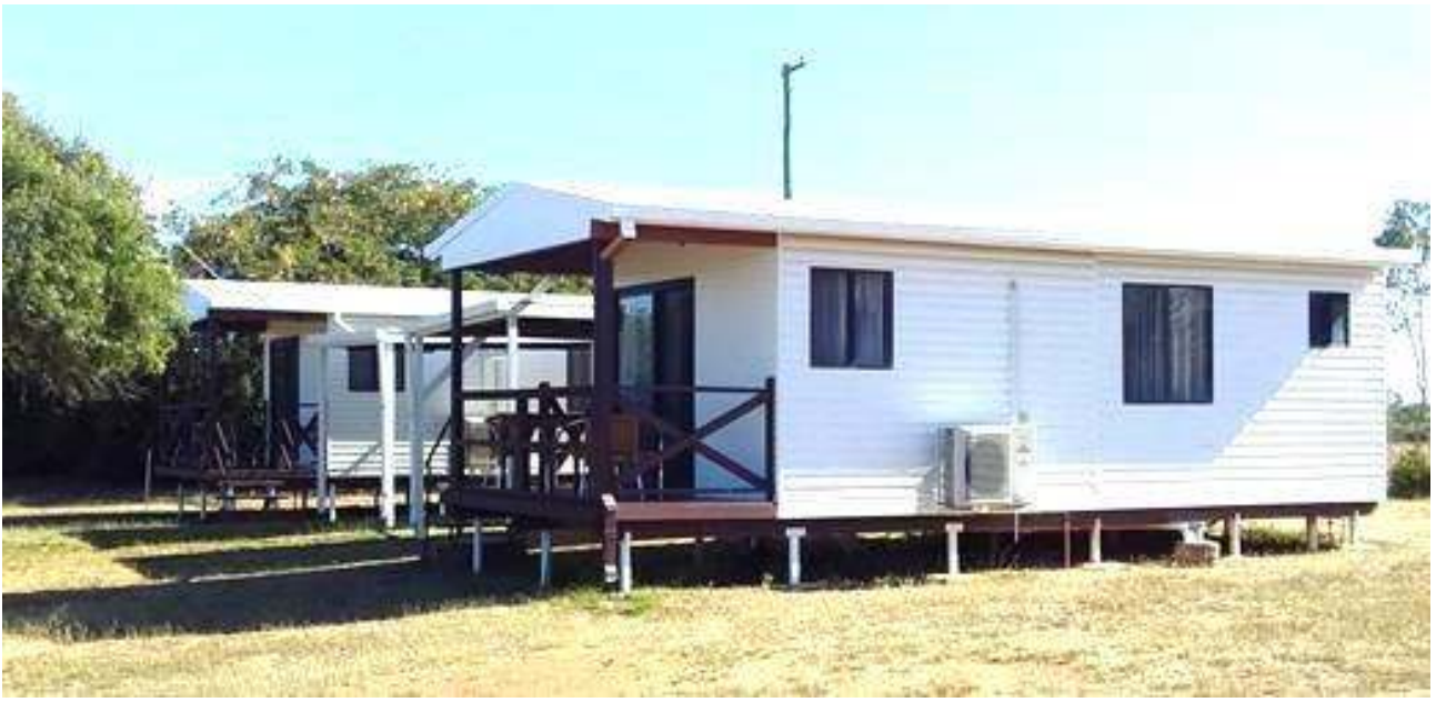
Figure 18a: Refurbished accommodation cabins at Top Camp
