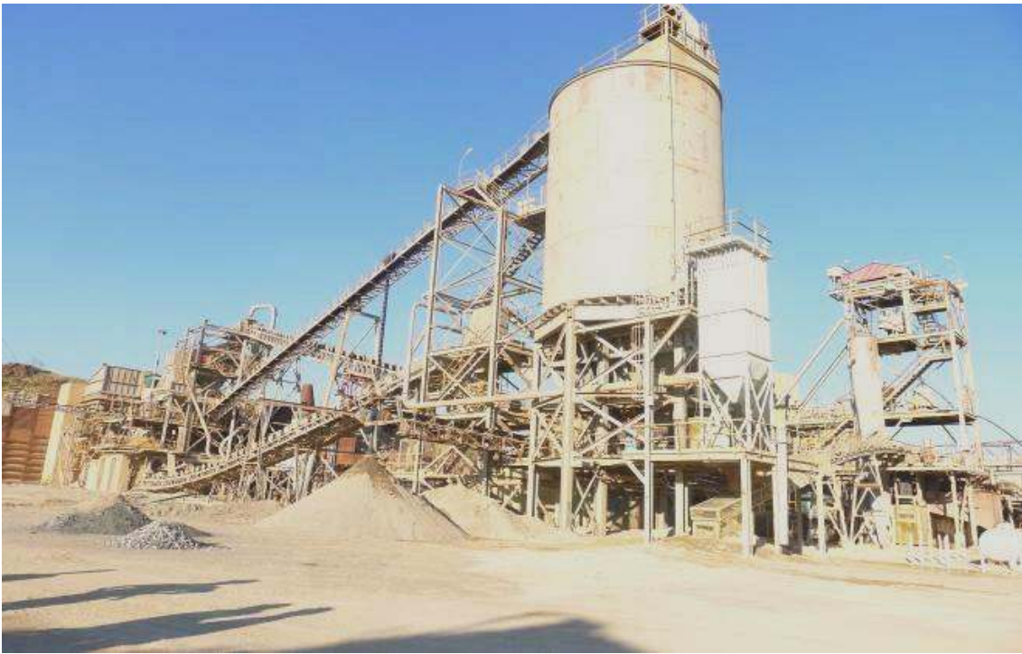
Figure 3: Bamboo Creek Processing Plant
