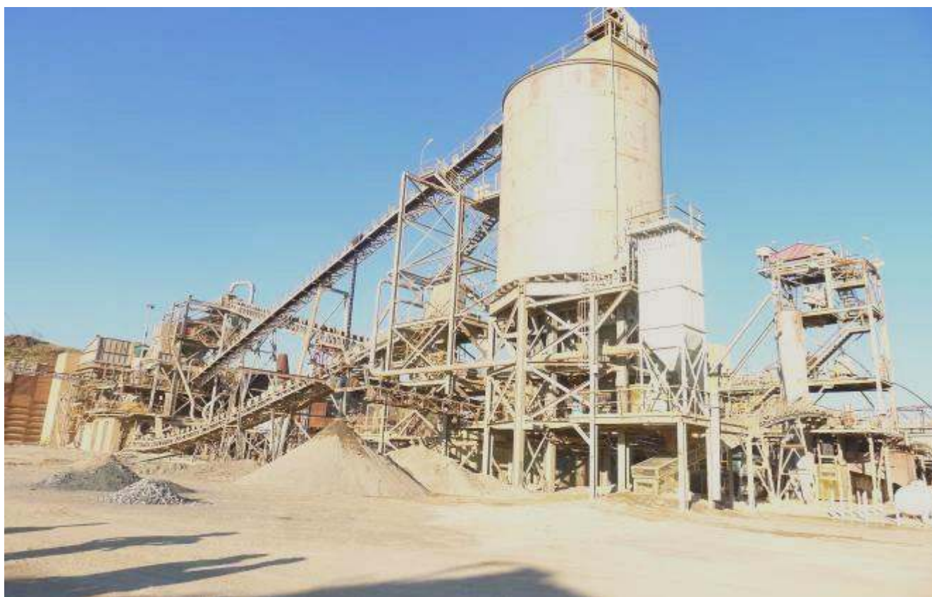
Figure 14: Bamboo Creek Processing Plant
