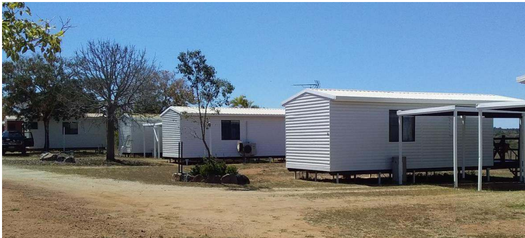
Figure 7(b): Refurbished accommodation cabins at Top Camp
