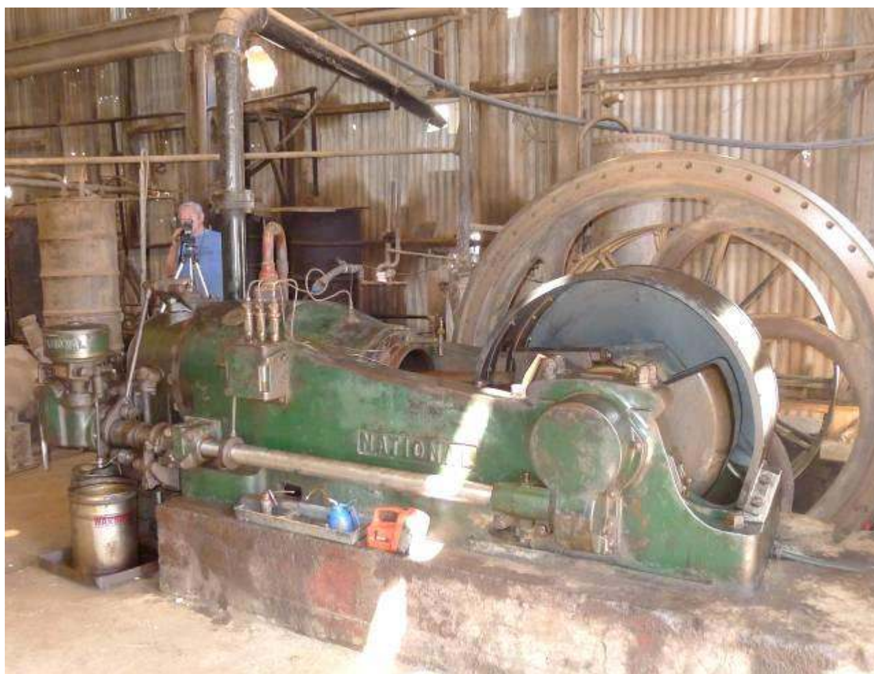
Figure 12: Comet Gold Mine National Diesel Power Engine
