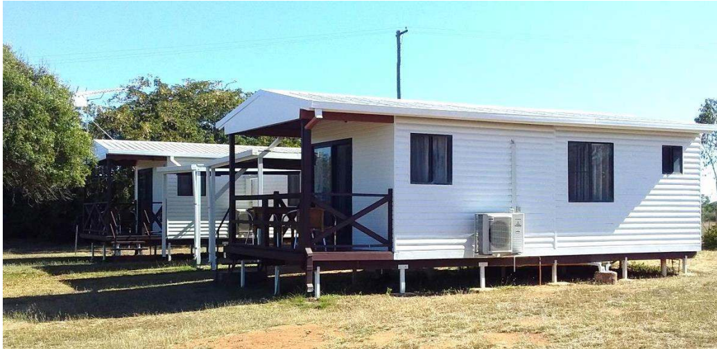
Figure 7(a): Refurbished accommodation cabins at Top Camp
