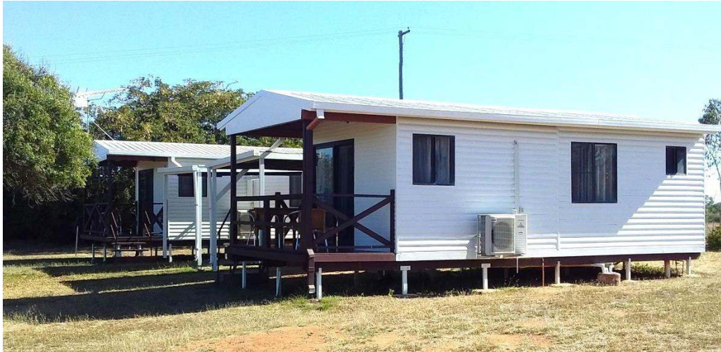
Figure 13(a): Refurbished accommodation cabins at Top Camp
