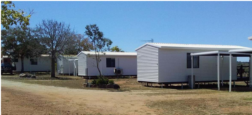
Figure 13(b): Refurbished accommodation cabins at Top Camp
