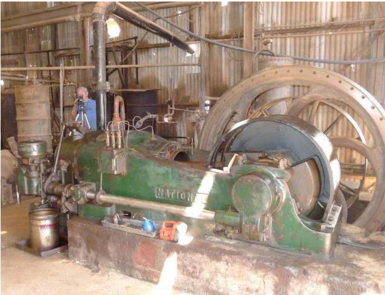
Figure 18: Comet Gold Mine National Diesel Power Engine
