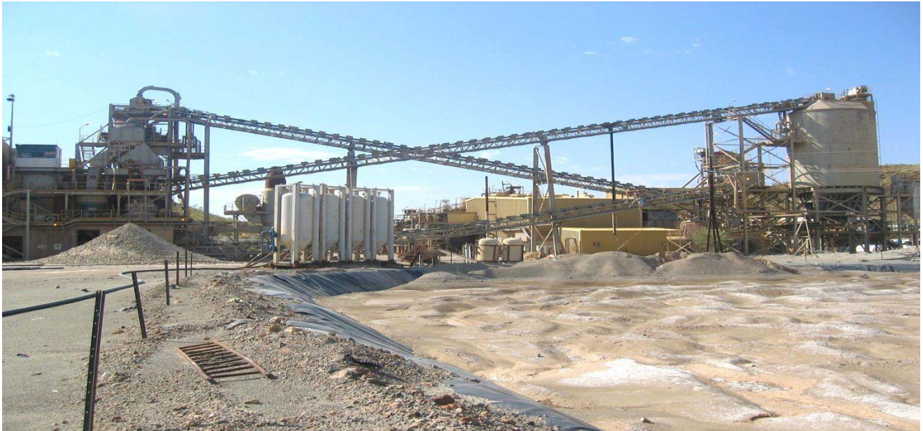
Figure 21: Bamboo Creek Processing Plant
