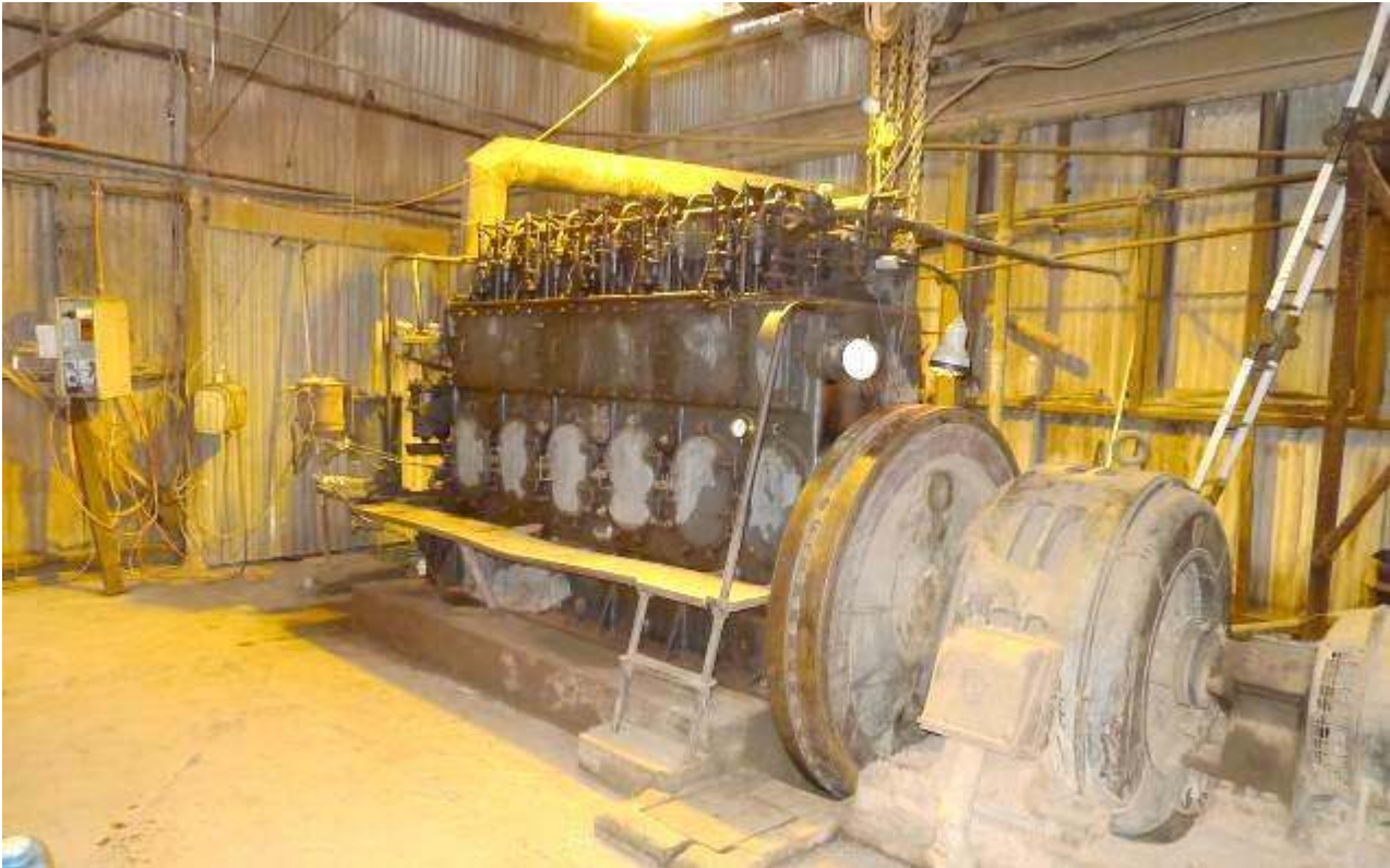
Figure 17: Comet Gold Mine Ruston Diesel Power Engine.
