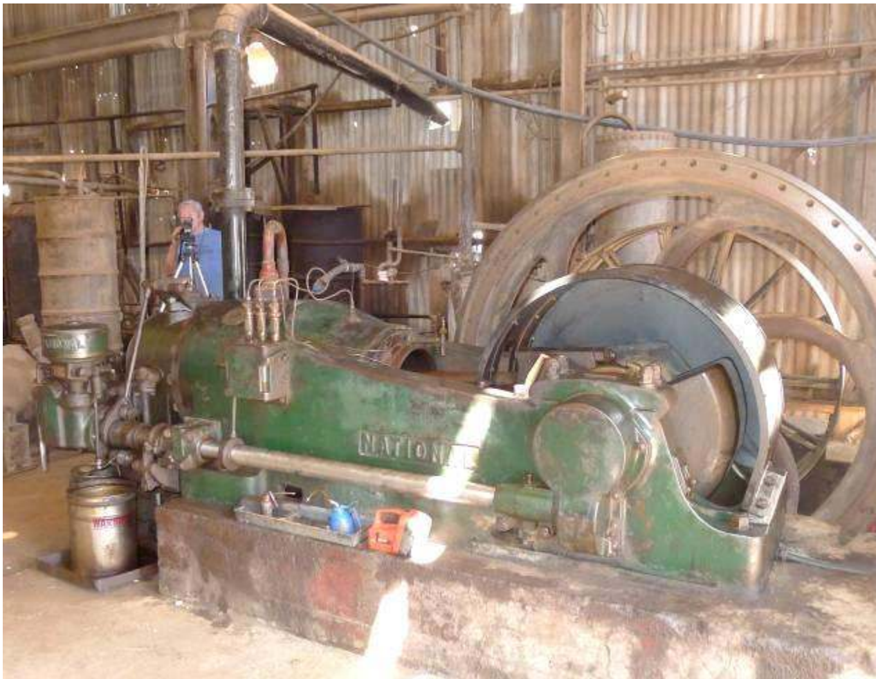
Figure 18: Comet Gold Mine National Diesel Power Engine.
