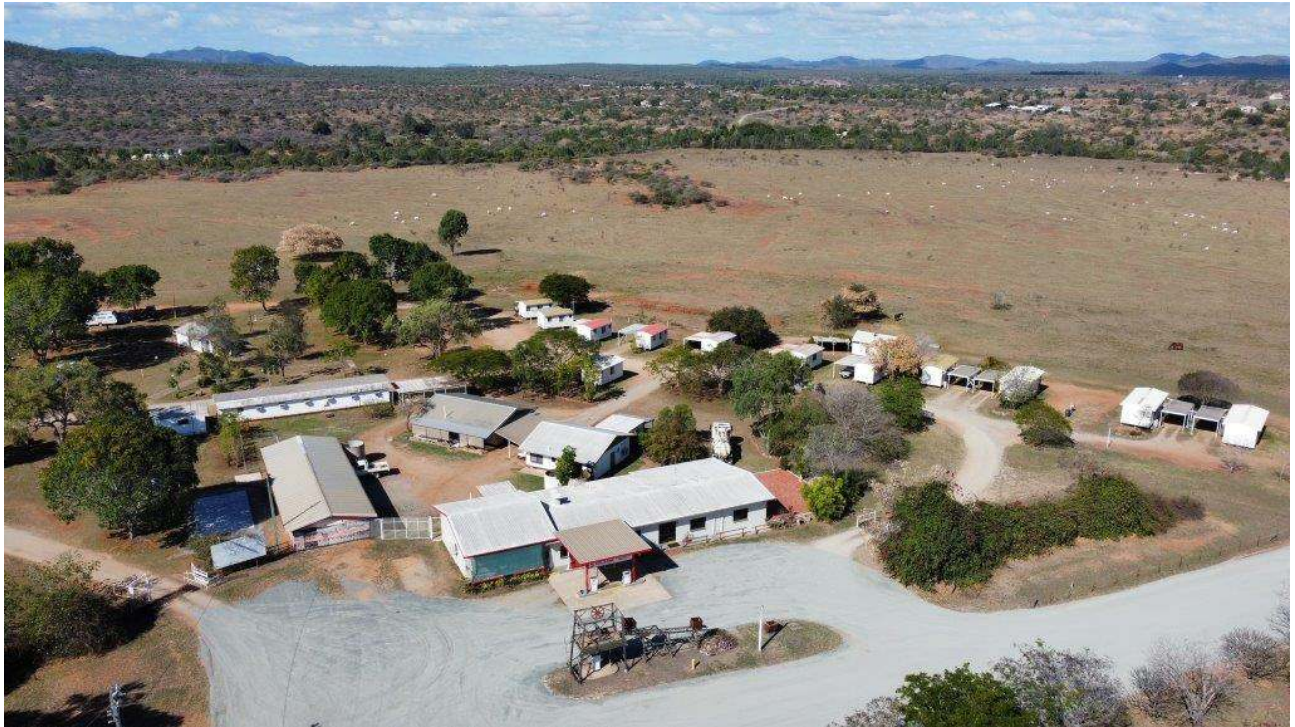
Figure 12: Aerial view of Haoma’s Top Camp, Ravenswood, Queensland.
