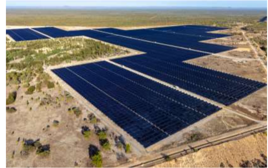
Kidston 50MW Solar Project
