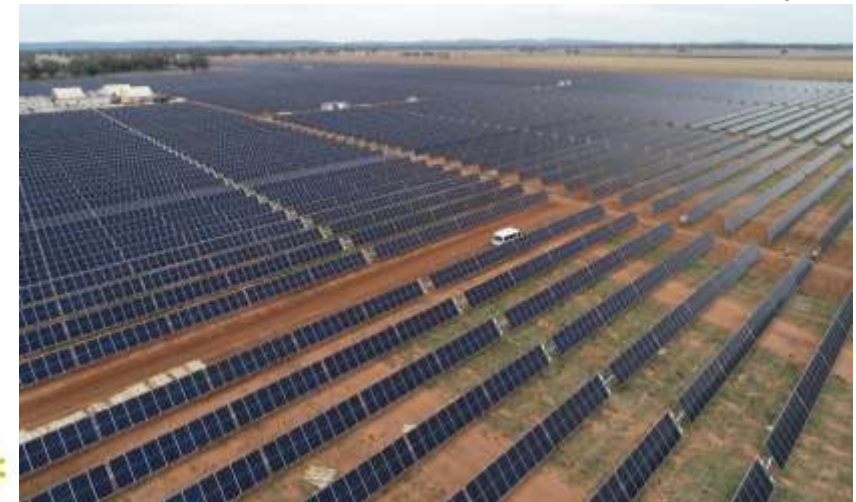
Jemalong 50MW Solar Project
