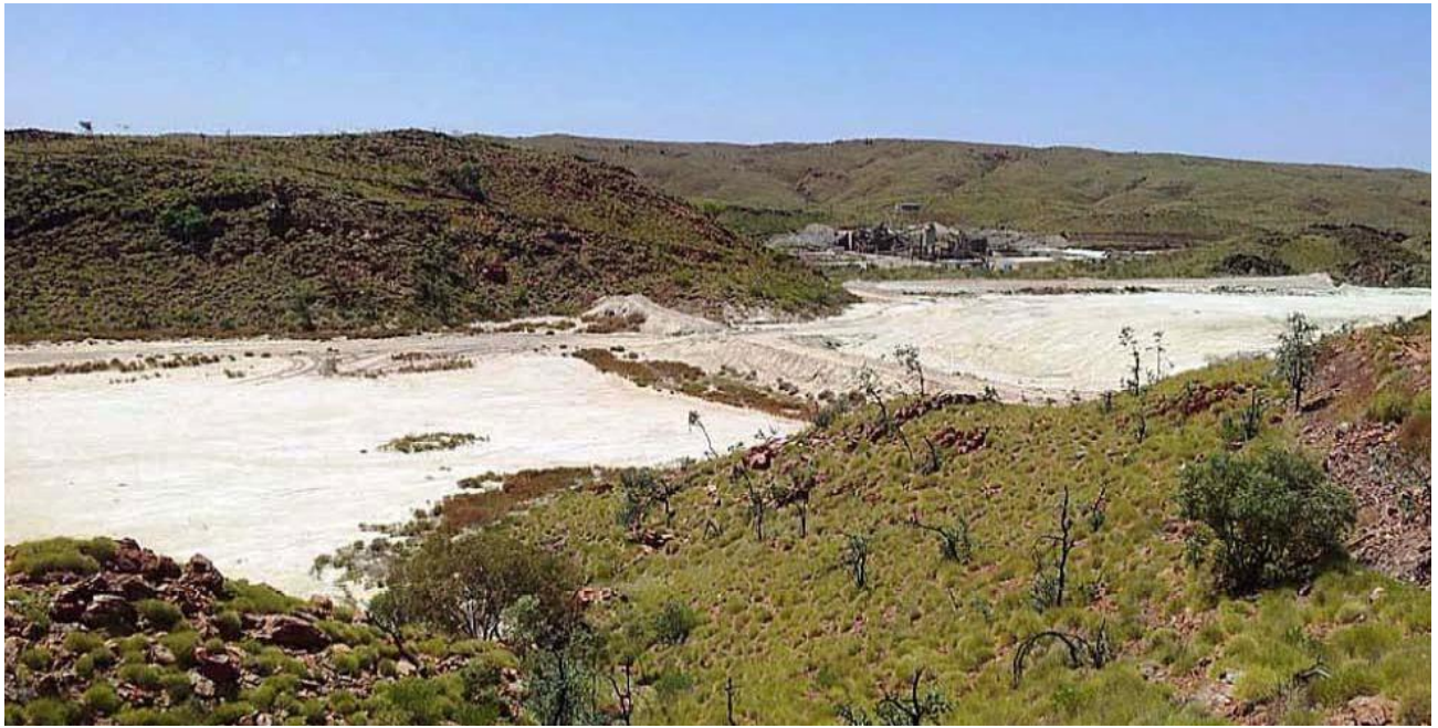
Figure 20: Bamboo Creek Tailings Storage with Bamboo Creek Processing Plant in background
